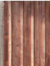
Expressed cover strips at board joints
