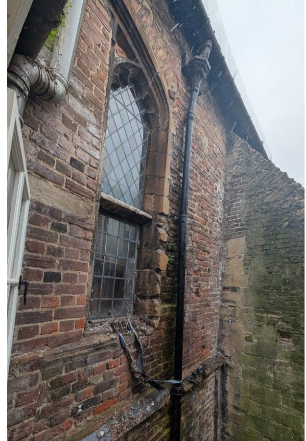
Historic filled in window to be reopened to form doorway to extension
