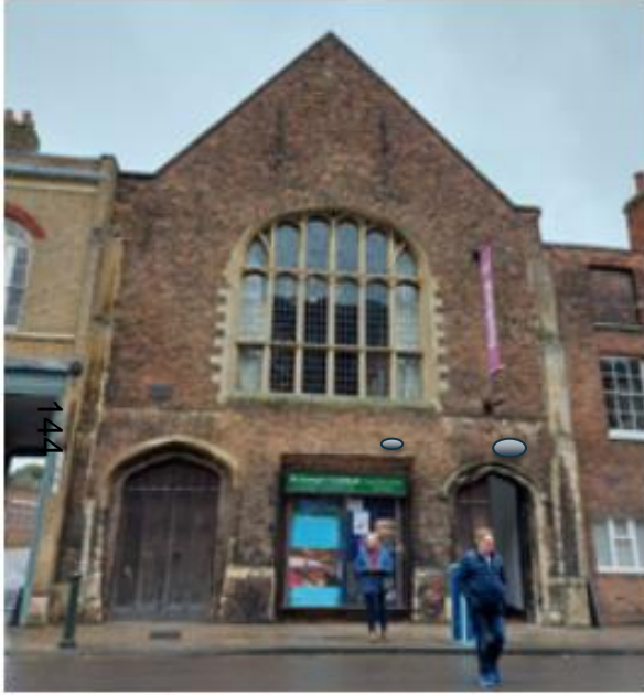
Existing Guildhall facade to King Street
