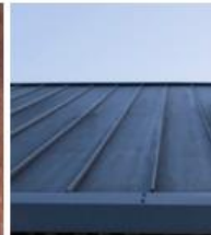
Zinc standing seam roofing
